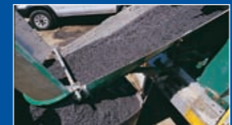
2 AFTER SUFFICIENT MIXING, COLOURED CONCRETE IS DISCHARGED FROM CONCRETE TRUCK
