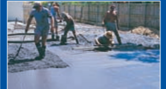
3 COLOURED CONCRETE IS SCREEDED AND FLOATED
